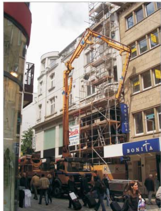
Concrete works shortly before the assembly of the new facade.
