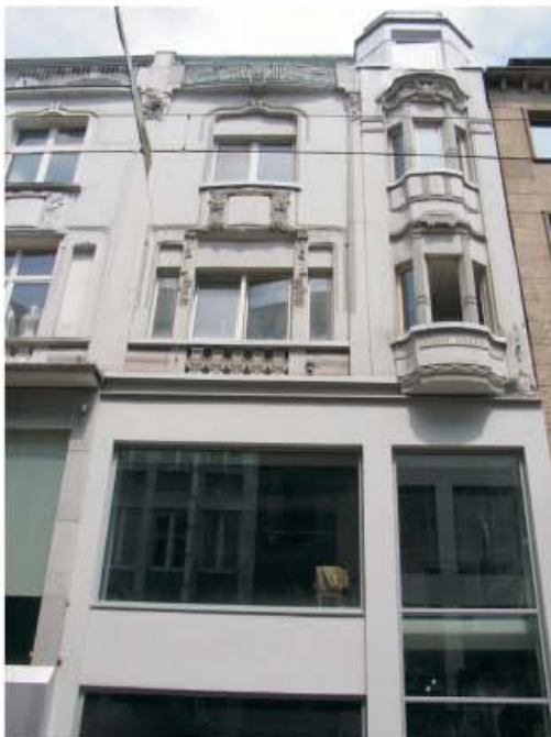
The property at the day of handover to the tenant.
